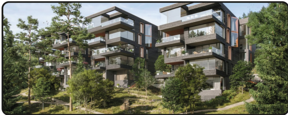
Fig. 1. The case study using one of these apartment buildings in Oslo, Norway [9].
