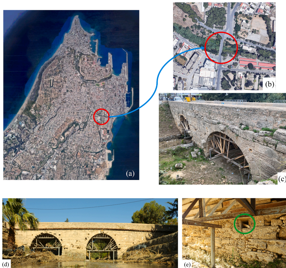
Fig. 2. (a) Rhodes Island in Greece and location of the Roman bridge, (b) top view of the Roman bridge, (c) and (d) Roman bridge from different views, and (e) holes in the central pier with erosion.
