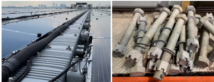
Fig. 6. Connections between floating modules (left) and nylon bolts for the connectors (right).
