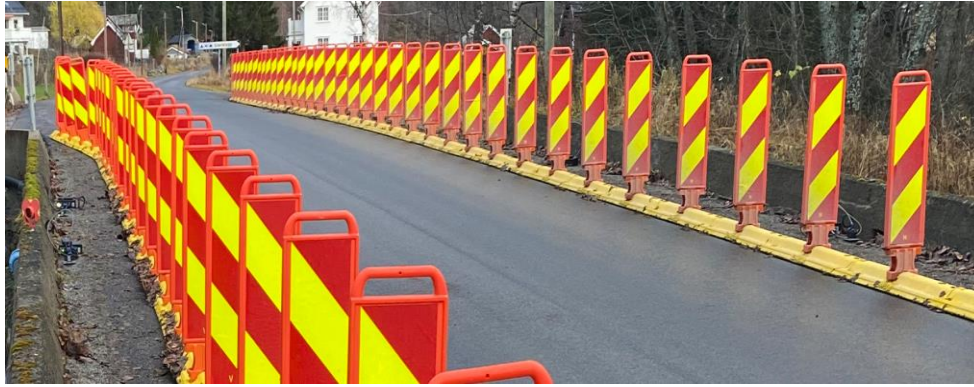
Figure 42: OMAway sensors installed on each side of the concrete bridge
