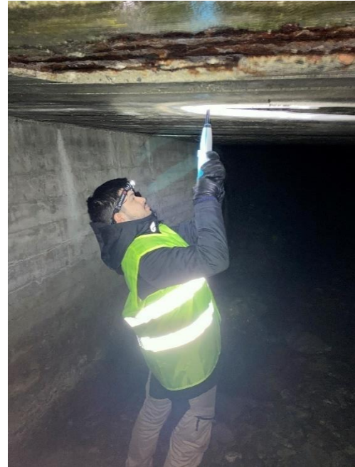
Figure 23: Rebound hammer performed in situ
