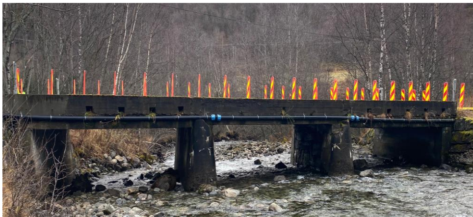
Figure 2: Øvre Kvamme bridge in Lærdal at time of inspection
