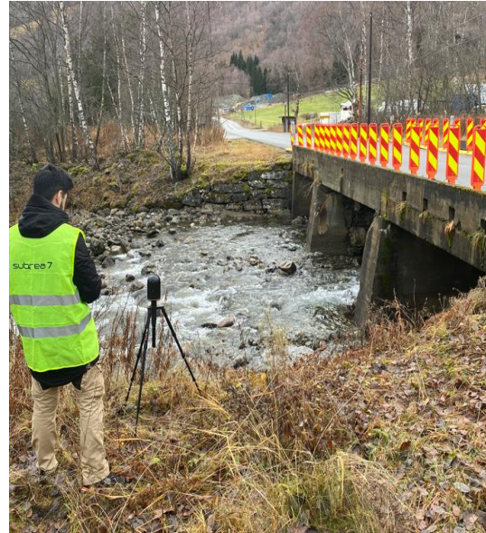
Figure 39: 3D scanning performed in situ
