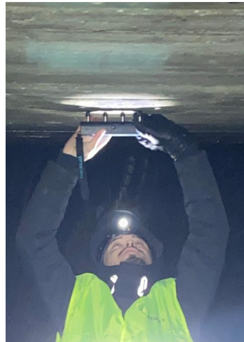
Figure 34: Concrete resistivity instrument performed in situ
