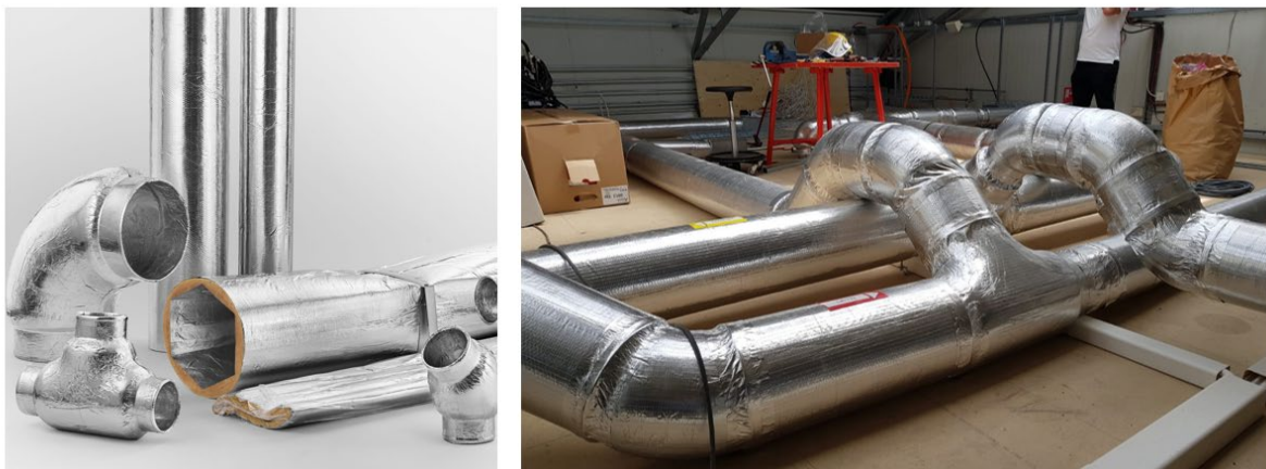
Figur 19: Climate recovery system [61]
