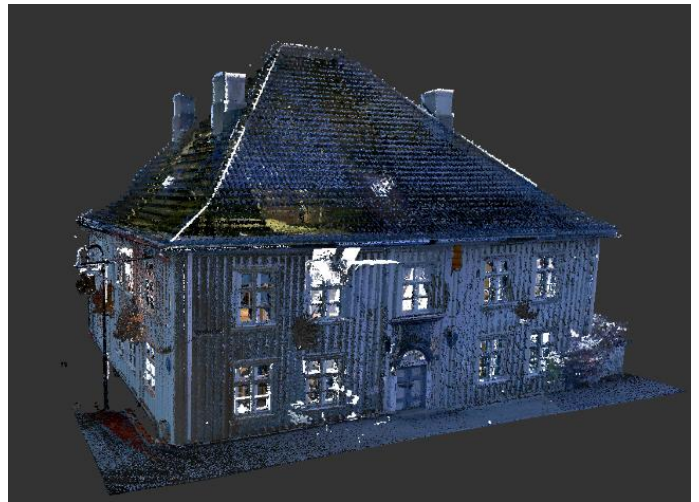
Figure 3 Point cloud of the old hospital building
