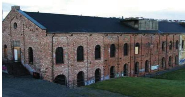
Figure 1: Case study- Industrial heritage building -PM5
