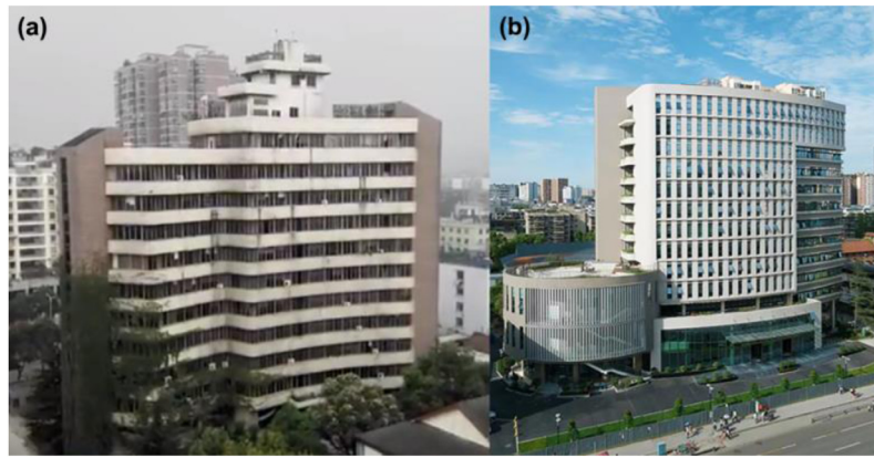
Fig. 2. Photos of the building before (a) and after (b) the retrofit.
