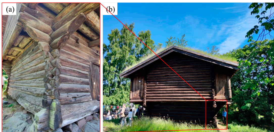
Figure 17. (a) Carpentry corner joint of the logs; (b) a heritage log house building in Tønsberg, Norway—Heierstad loft.
