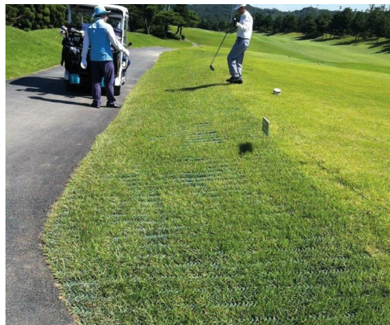
Bilde 6: Gressarmering langs vei (External Works)
