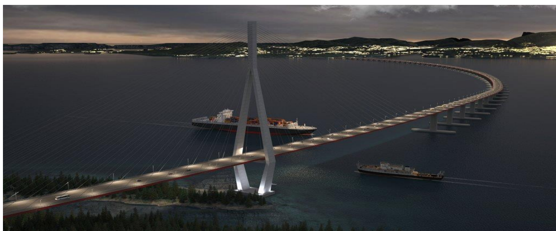
Figure 4.1. Curved floating bridge concept. Illustration by The Norwegian Public Roads Administration[42].
