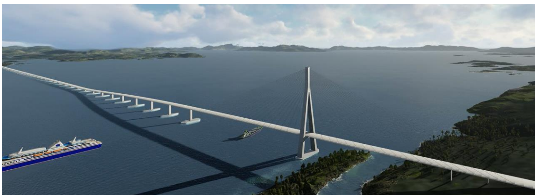
Figure 5.1 Straight floating bridge across Bjørnafjorden [45].
