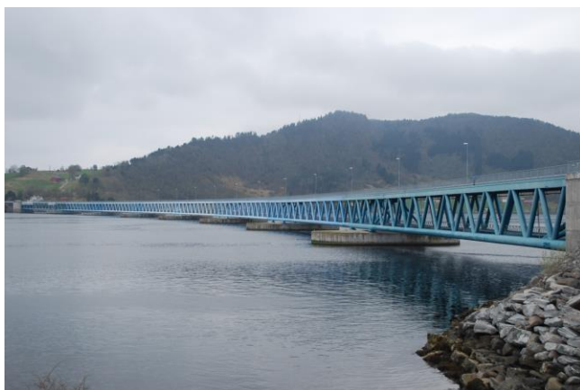
Bergsøysund bridge [11] - Picture [12]
