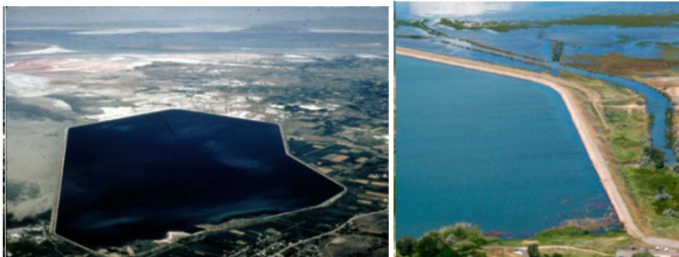
Fig. 3.3 Arthur V. Watkins dam oversikt (U.S. Department of the Interior Bureau of Reclamation, u.å., 1. avsn.)
