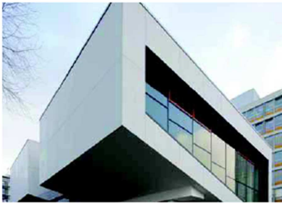
Façade panels on the lecture building at RWTH Aachen
