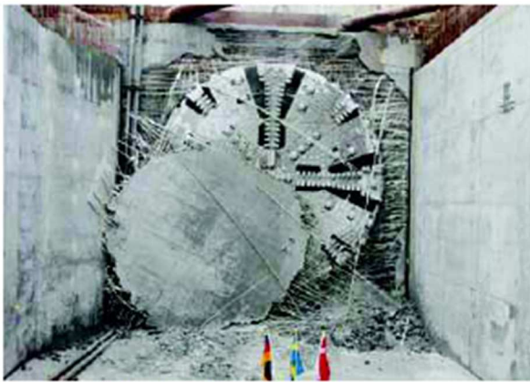
Central Station, City Tunnel Malmö, Sweden
