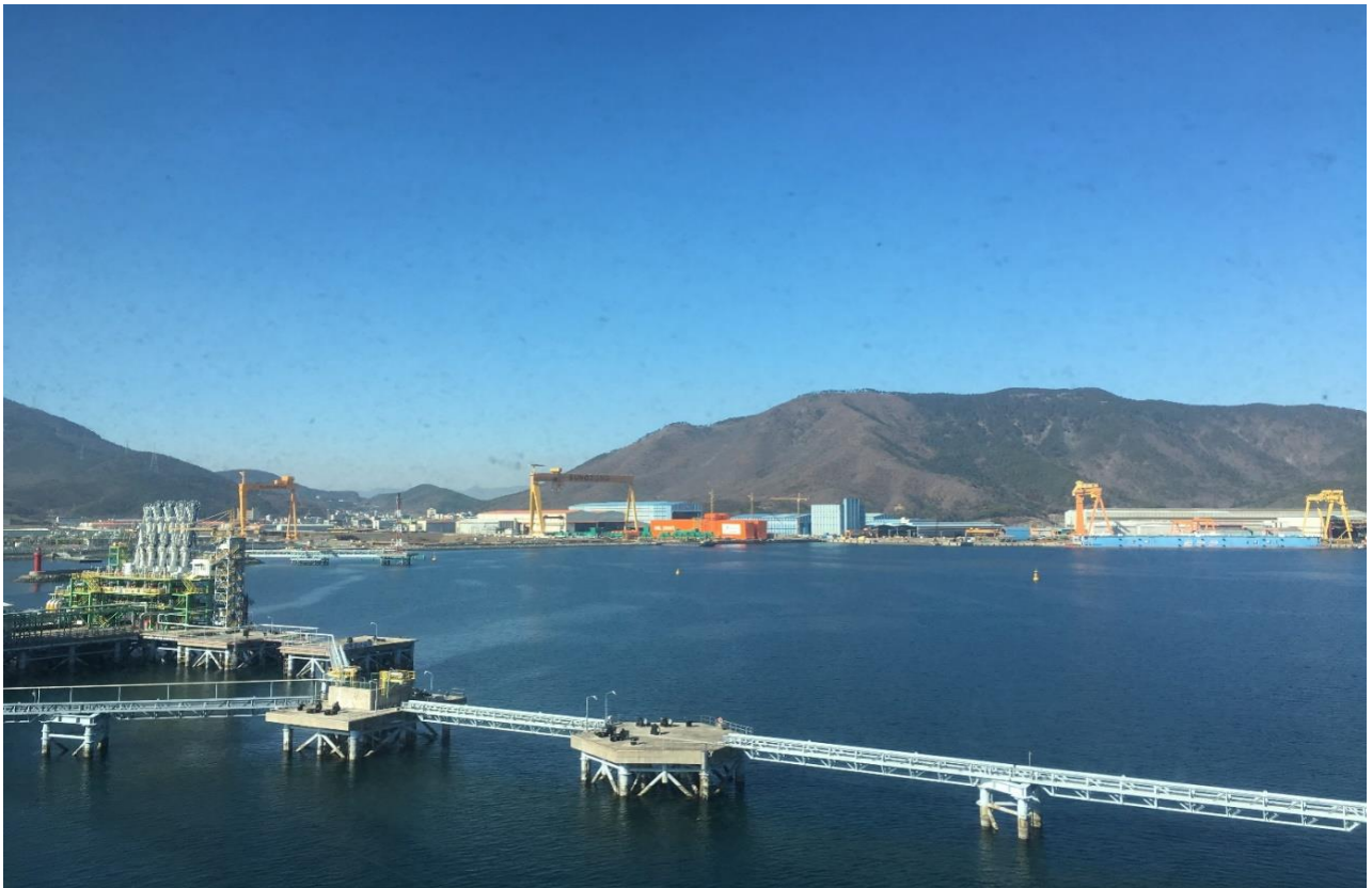
LNG terminal in South Korea, seen from aboard. Photo by author.
