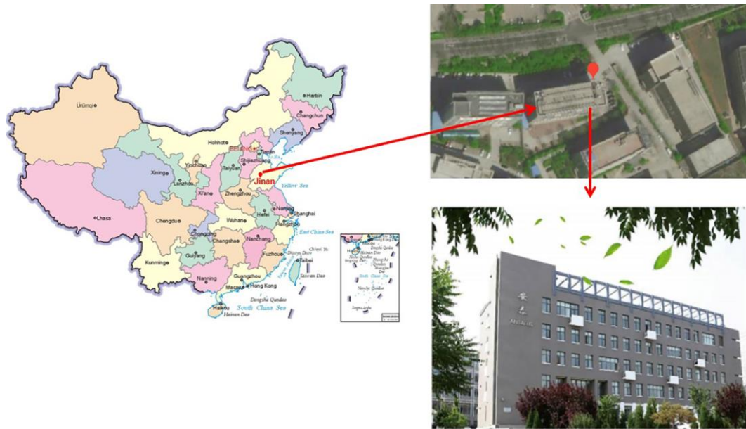
Fig. 4. The location and side view of the office building.
