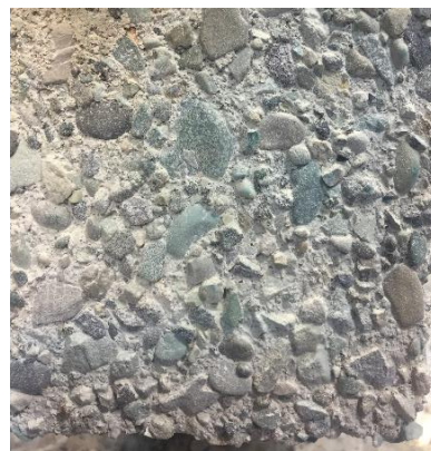
Figure 12. Visual inspection of OPC sample (100 × 100 mm) exposed to sulfuric acid after 6 months.
