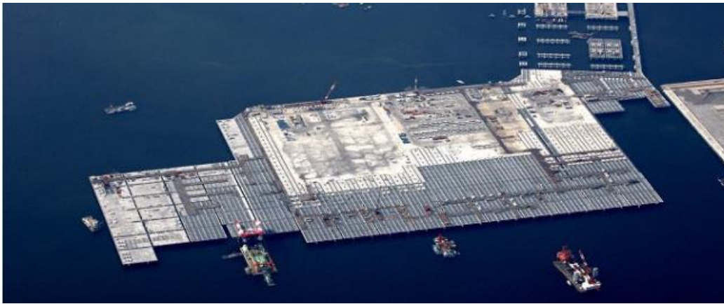
Figure 2.18:UHPFRC applications in the marine bridge (Extension of Haned airport) [65]
