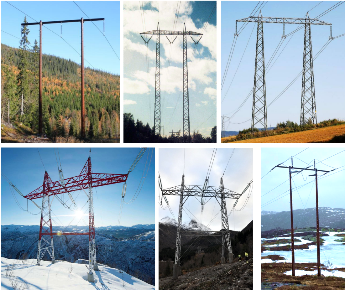
FIGURE 2.6. EXAMPLE OF H-PORTAL PYLONS IN NORWEGIAN POWER GRID [60]
