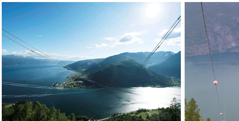
FIGURE 2.15. POWERLINE CROSSING FJORDS (A) 3350 M FJÆRLANDSFJORDEN POWERLINE [4] AND (B) 4570 M REFSDAL – FARDAL POWERLINE OVER SOGNEFJORDEN [72]
