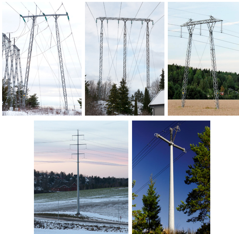
FIGURE 2.5. EXAMPLE OF GUYED STEEL TOWERS AND SELF SUPPORTING STEEL POLES [60]
