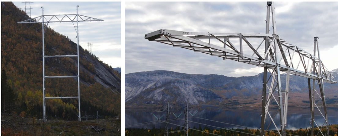
FIGURE 2.22. STATNETT'S AND EFLA'S ALUMINUM TOWER FOR 420kV POWERLINE [80]
