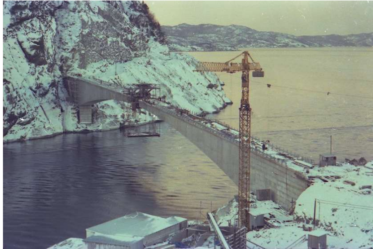
Figure 7: Osstrupen Bridge during construction in 1976 3
