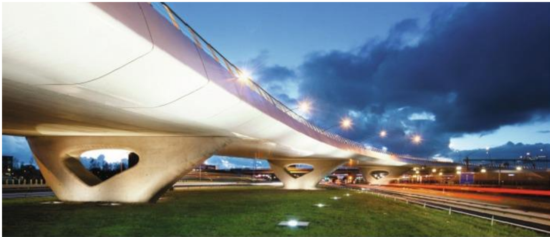
Figure 2.5: Fly-over Waarderpolder bridge in Netherland with FRP edge elements [29].
