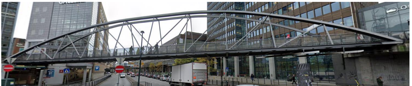
Figure 3.1: Picture of the pedestrian bridge in Oslo
