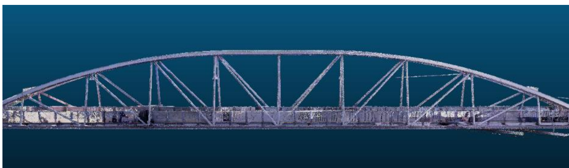
Figure 1.1: The bridge that is curved in two directions
