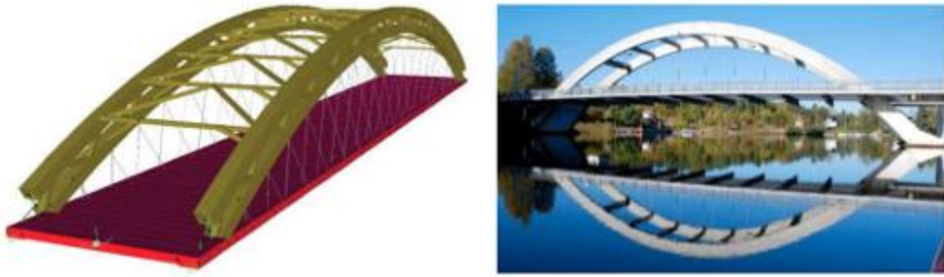
Figure 53: Left) Oppstadåa network arch bridge with timber arches, Right) Vippsa bridge with concrete arches [69]
