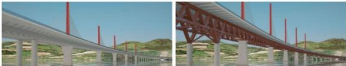
Figure 57: Design suggestions for the new Mjøsa bridge. Left) Concrete deck. Right) Timber trusses [71]
