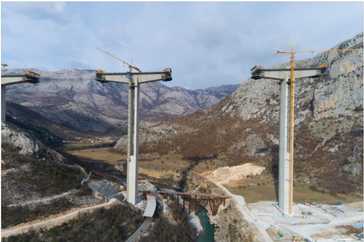
Figure 16: Balanced concrete cantilever bridges during construction [22]
