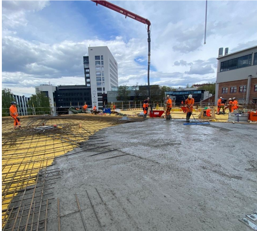
Figure 2. Post-tensioned slab cast at Gullhaug Torg 2A
