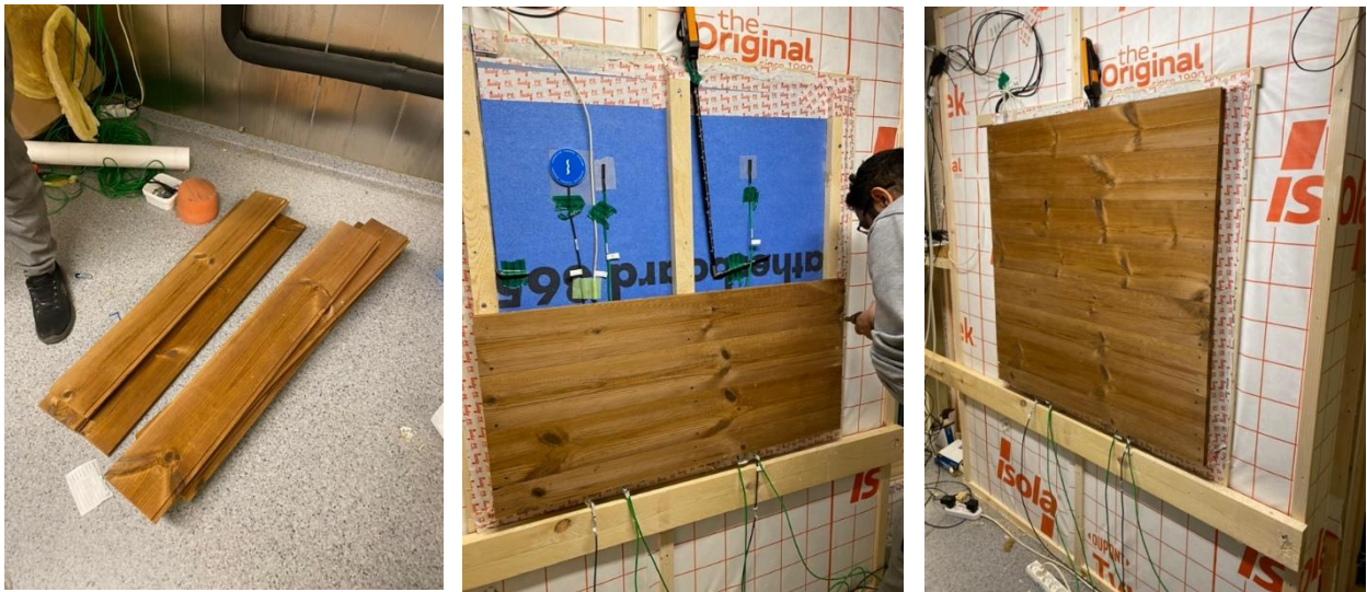
Figure 27: Mounting of the wooden cladding.
