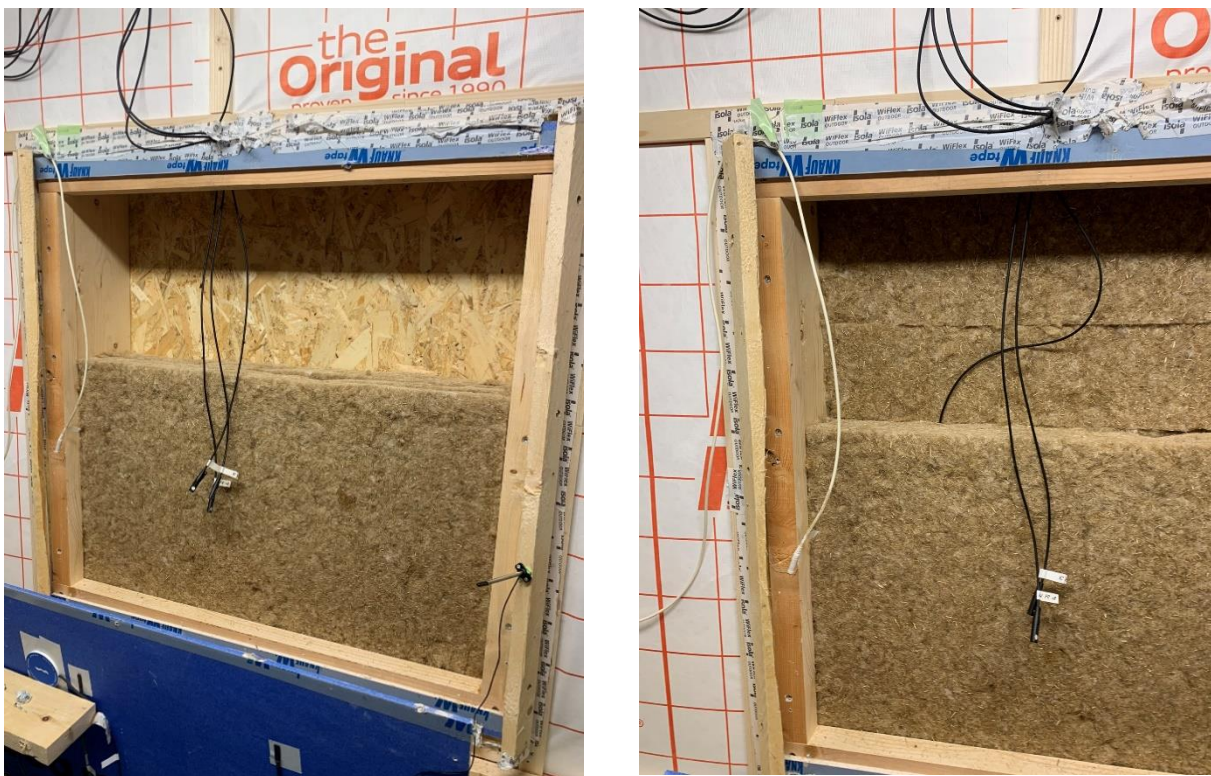
Figure 25: Mounting of flax fibre and Onset S-THC-M008 sensors.
