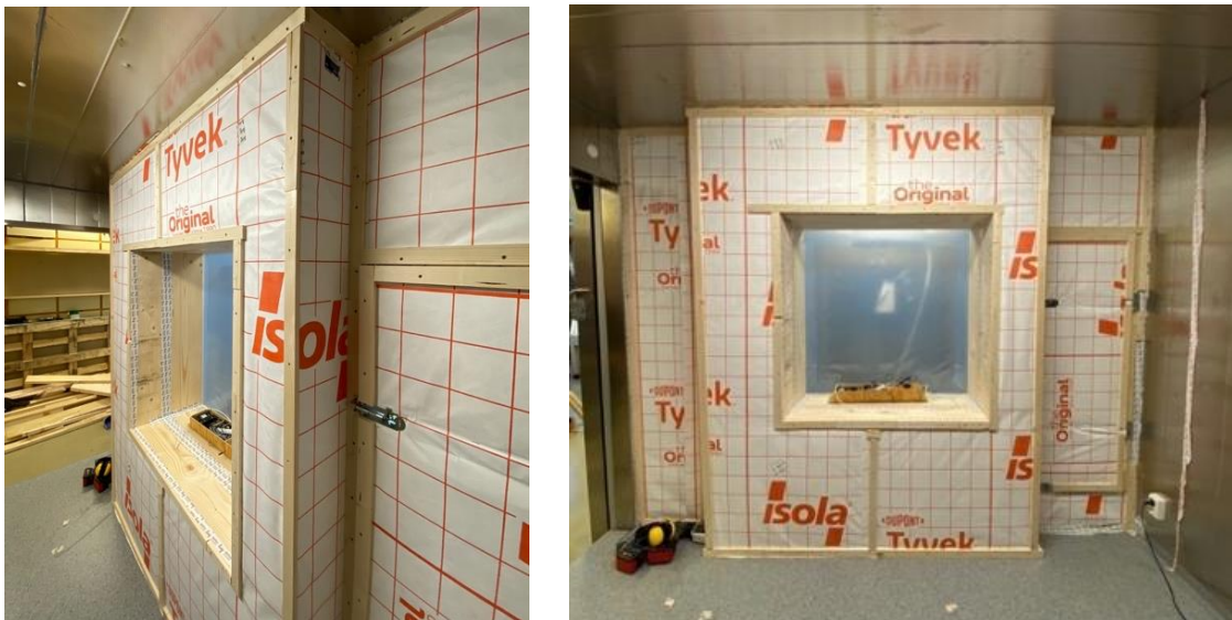
Figure 10: Separating Wall - Finished product
