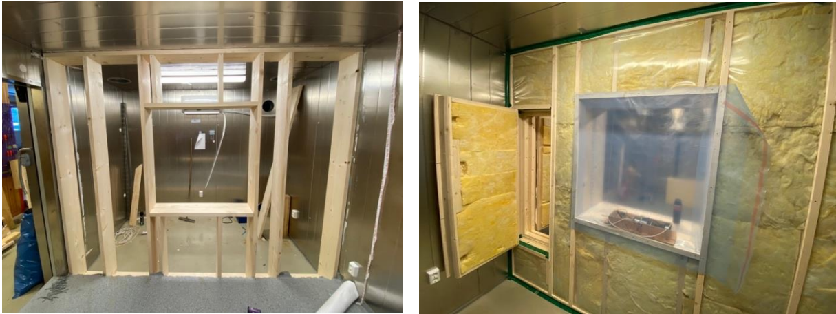
Figure 9: Separating Wall - Building process
