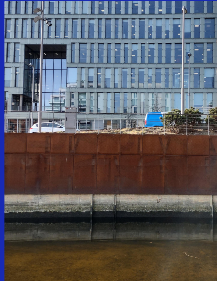
Figure 3: Harbor front in Oslo harbor, by the author, 2022.
