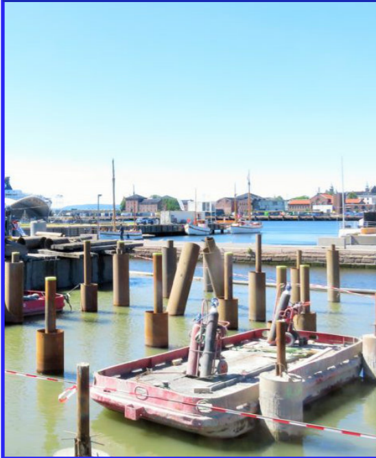
Figure 11: Steel pillars in Oslo harbor, by Veidekke, 2016, https://munch.veidekke.no/2016/06/20/kompetent-fundamentprodusent/ .
