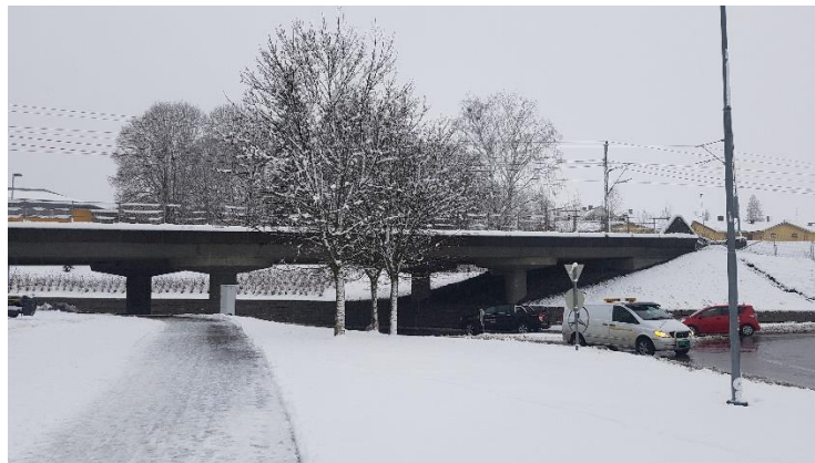
Figure B.1. Stange railway overpass.
