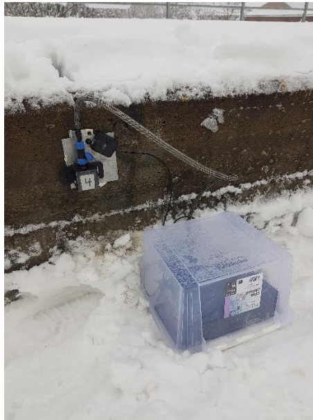
Figure 19. Accelerometer and datalogger installation.
