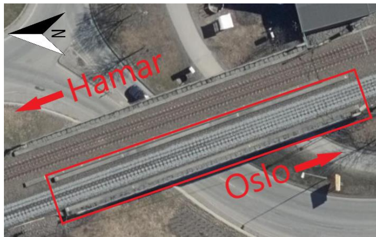
Figure 6. Aerial photo of Stange railway overpass [34].
