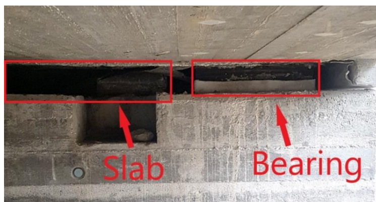
Figure 40. Concrete slab underneath deck extensions in relation to bearing.
