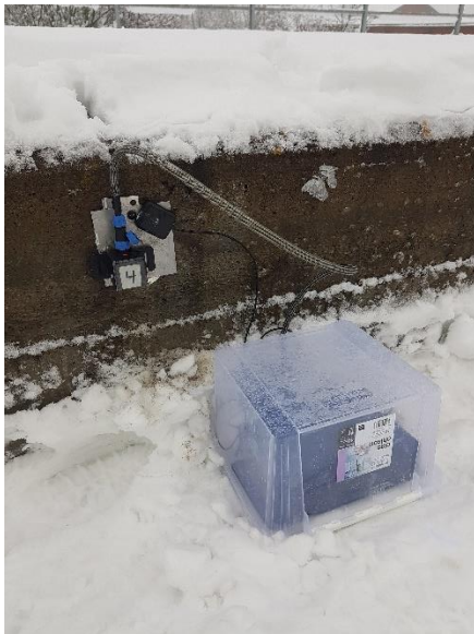
Figure B.2. Datalogger and accelerometer setup.
