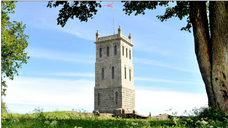
Figure 3 The Slottsfjell tower [32]
