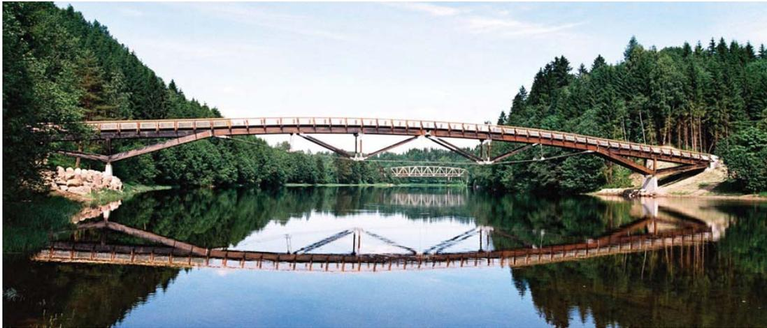
Figure 1: The Kjærø Bridge has a total span of 132m and a free span of 92m across the Numedalslågen River in Lardal, Norway. Photo: Lisbeth Michelsen
