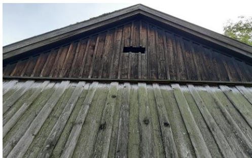
Fig. 4. Microclimatic conditions have a strong impact on the discolouring as well as the development of lichen on coating's surface.
