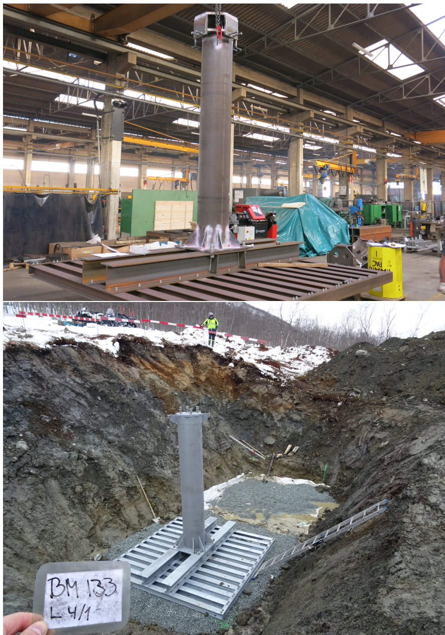
Figure 1.2: Steel foundation
