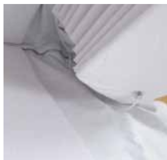
ill. 56: Folding details and fastening to the wall
