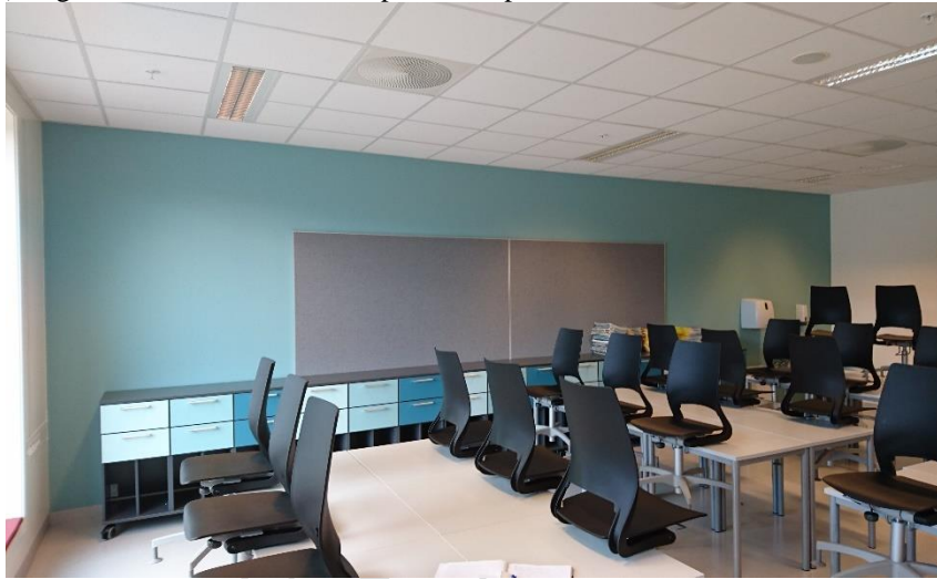
Fig. 2. The test room at Fernanda Nissen School, Oslo. All of the education rooms have mixing ventilation with similar air inlet and outlet as the test room. (Photo: SINTEF).
