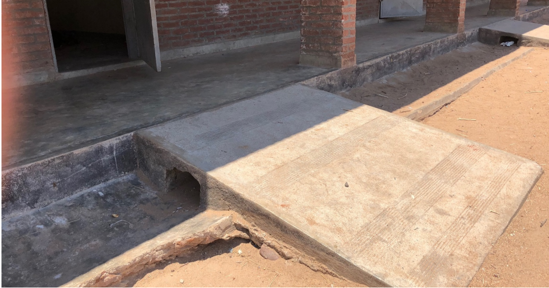
Photo 9, School 2 Malawi. Example of ramp.
