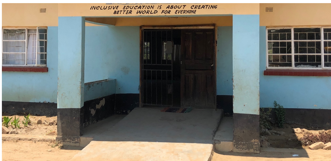
Photo 8, School 2 Zambia. Example of a well-designed ramp going all the way to the door.
