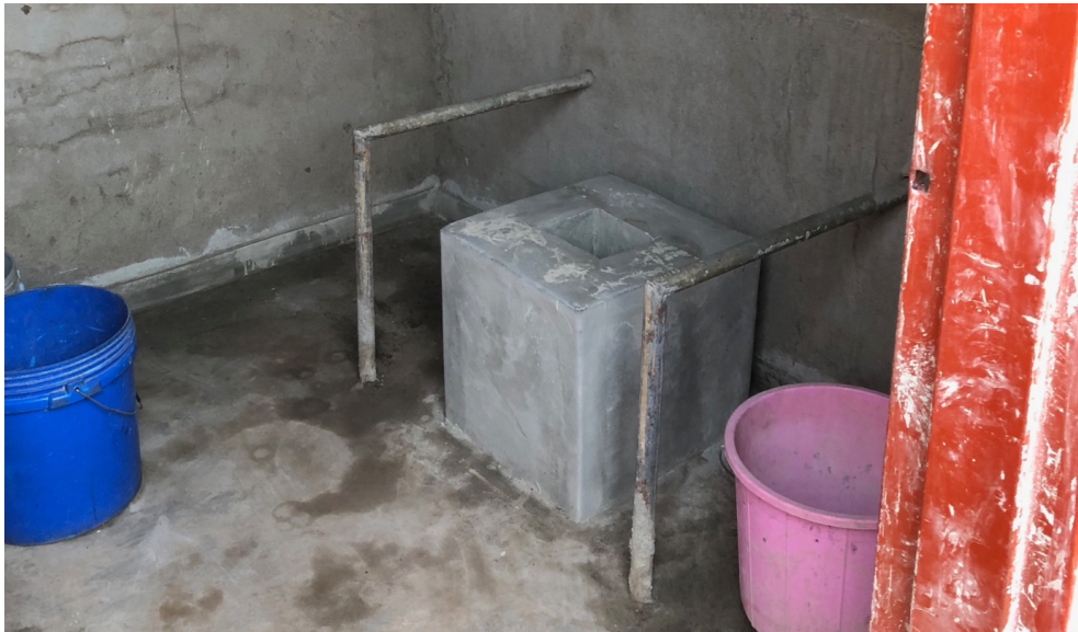
Photo 13, School 3 Malawi. Toilet facilities.
