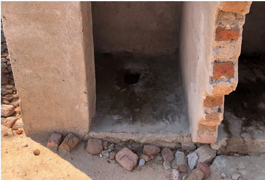
Photo 12, School 2 Malawi. Toilet facilities.
