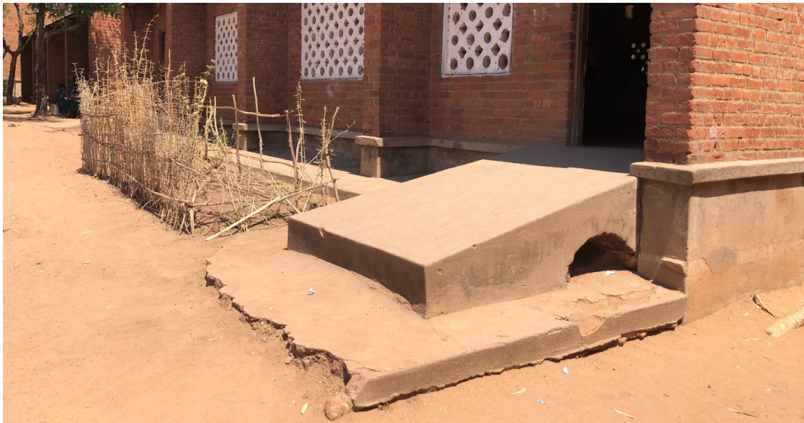
Photo 10, School 2 Malawi. Example of ramp.
