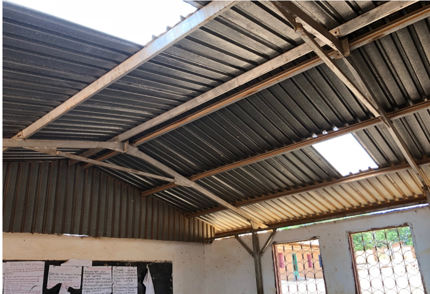
Photo 6, School 1 Malawi. Transparent roof panels.
