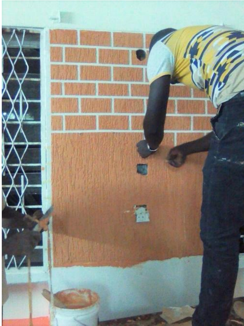
Figure:5 Lecturer demonstrate to the learners how to produce the stone finish technique.
