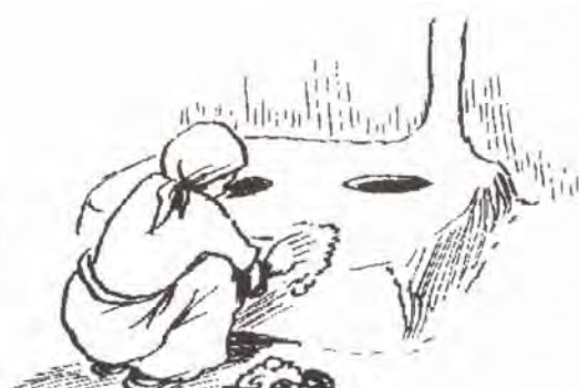
Figure A2.3 Filling in the crack with wet mud
