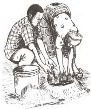
Figure 5.36 Mixing clay and sand with water
