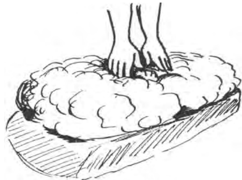
Figure 5.27 Heaping the mud balls
