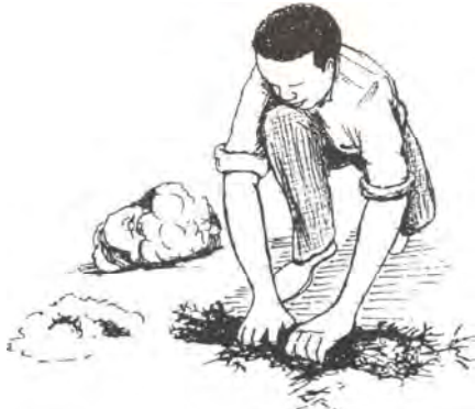
Figure 5.38 Rolling mud to form long pieces
