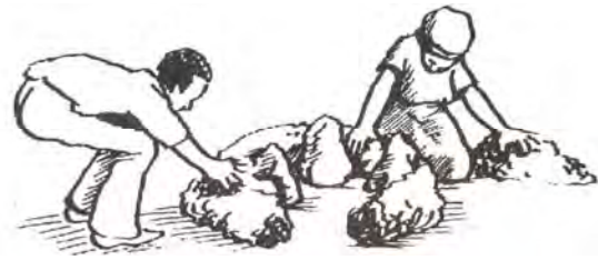
Figure 5.97 Smearing mud around the three stones
