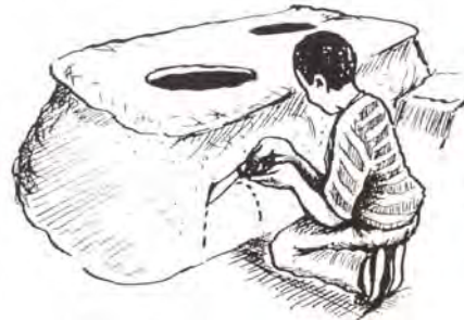
Figure 5.31 Cutting out the door
