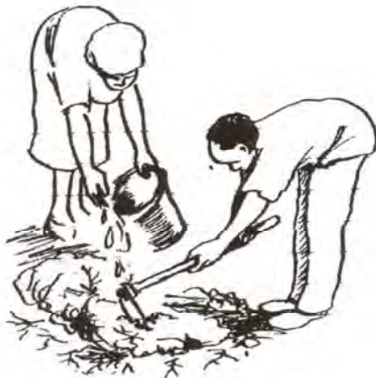
Figure 5.58 Mixing mud with water
