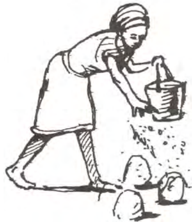
Figure 5.96 Sprinkling water on the stones
