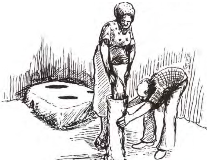
Figure A1.8 Removing the stem from the mud pipe
