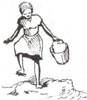
Figure 5.100 Mixing soil with water
