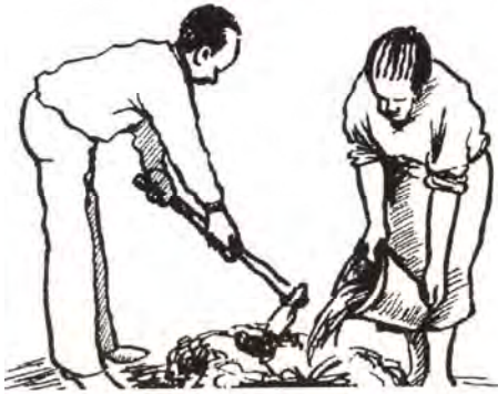
Figure 5.72 Mixing soil with water
