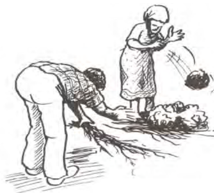
Figure 5.37 Spreading grass and throwing mud balls
