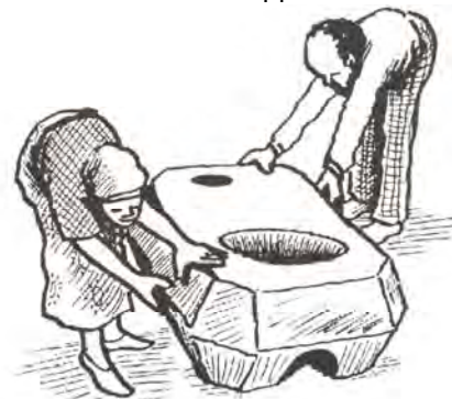
Figure 5.43 Fixing the top of the stove
