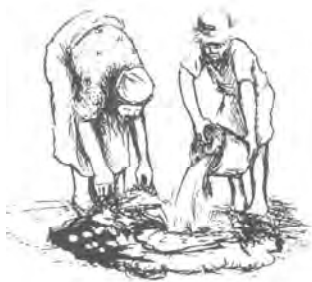
Figure 5.6 Mixing soil and water
