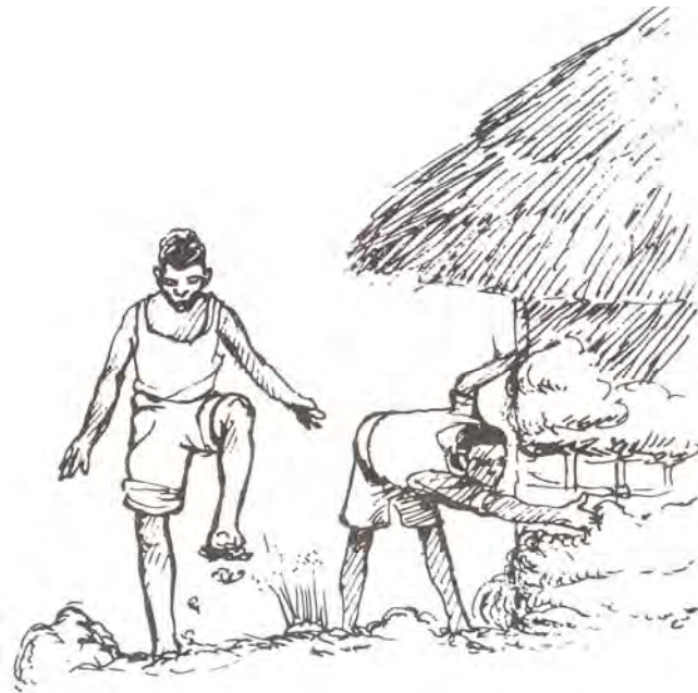
Figure 1.4 The walls of most houses in E. Africa were built of mud
