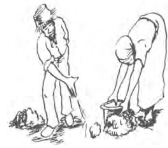
Figure 5.8 Packing mud around the sufuria
