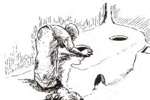
Figure A2.5 Filling in the crack
