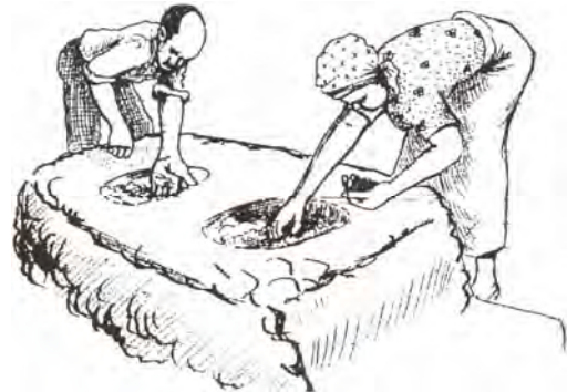
Figure 5.29 Scooping out mud to create fire chambers
