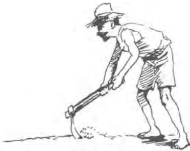
Figure 5.7 Levelling the ground
