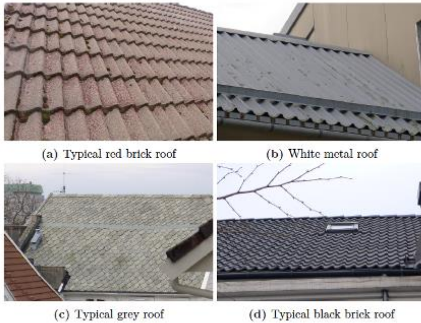
Figure 9: Types of roofing material in the Bryggen catchment area.
