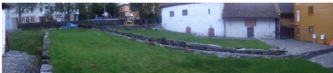
Figure 13: Impression of the treatment train with rainwater garden (under construction, left) and grassed swales (in the middle) and permeable pavement (lower right). (photo: F. Boogaard)
