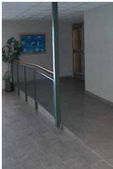
Figur v.18 Rampe – snublekant – i lobby
