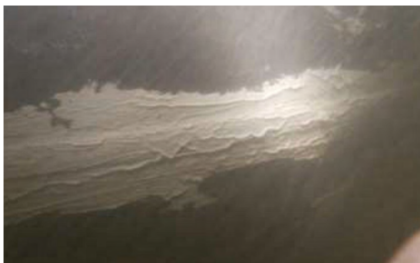
Figure 6.4: Resimac 208 Ceramic UW epoxy coating applied on underwater structure (U-CoatTechnologies 2023).
