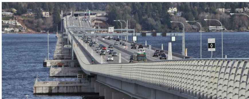
Figure 5: Evergreenpoint bridge (Wikipedia)
