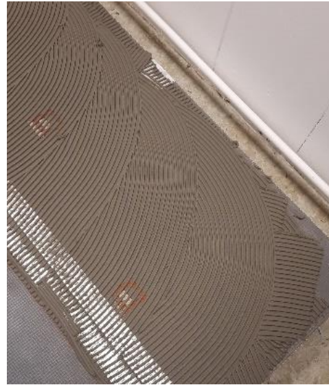
Figure 32 Random Tile Adhesive Grooves shown during Construction of EUT #4
