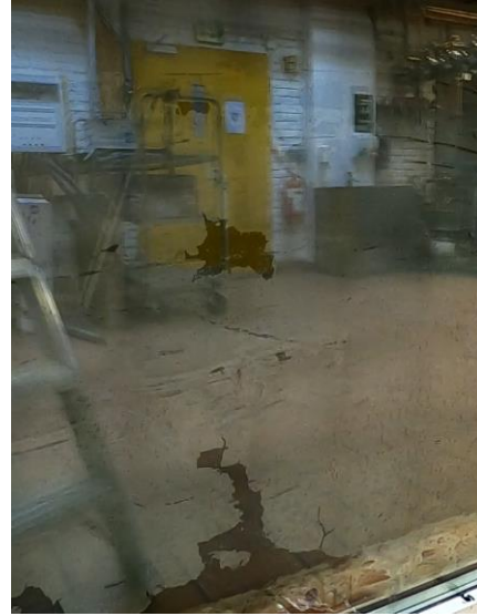
Figure 17 Water Exposure after 8 min – With Grout between the Tiles
