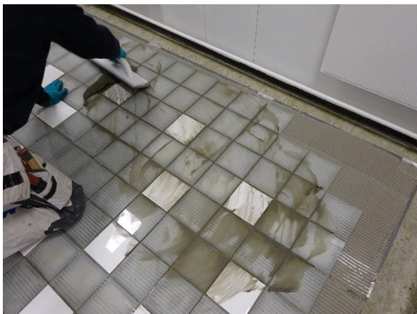
Figure 33 Grouting of EUT #1
