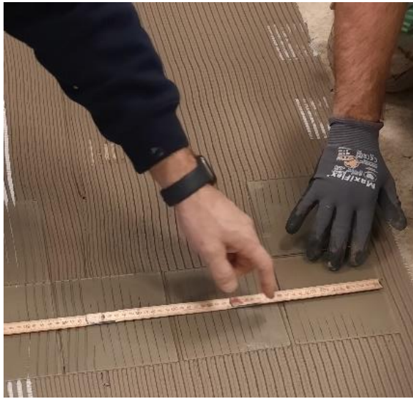
Figure 31 Horizontal Tile Adhesive Grooves, while Installing Tiles on EUT #1
