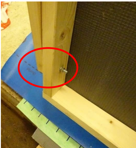
Figure 22 Support Legs Bolt Used for Stabilizing the Wall
