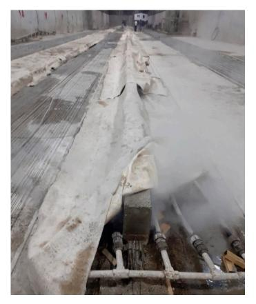
Figure 3. Curing of specimens via the steam method.
