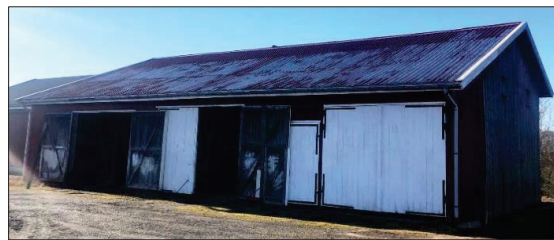
Figure 1. The first old barn from Sande.
