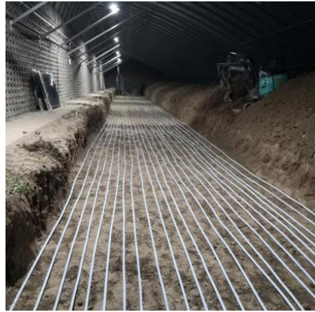
Figure 4. Horizontal heating pipe layout.
