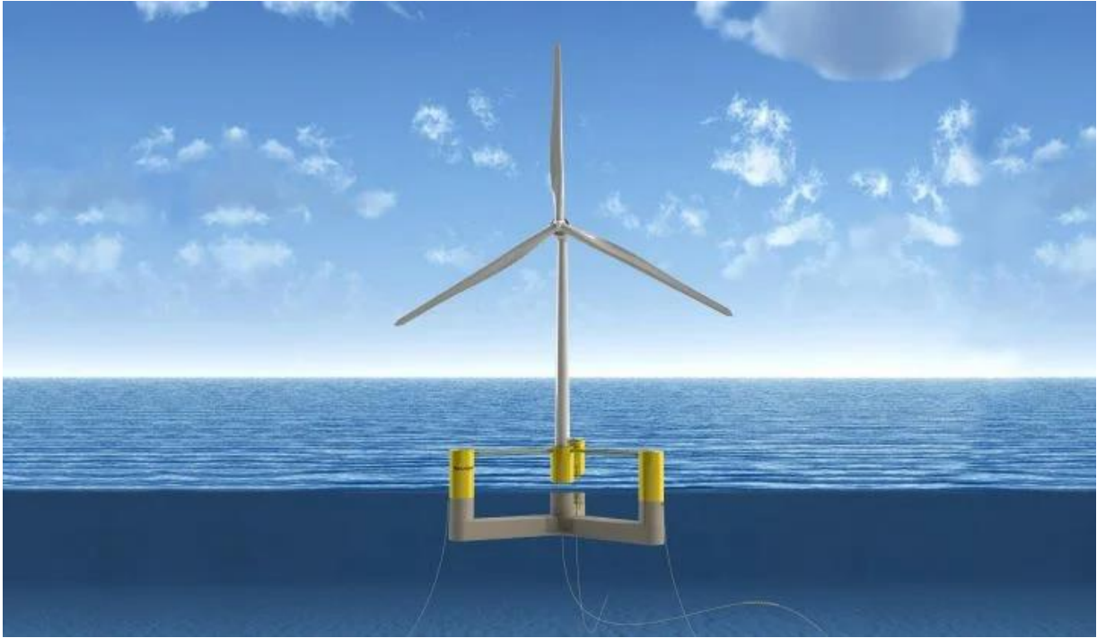
Figure 3.3: Semi-Submersible UMaine's University [80]
