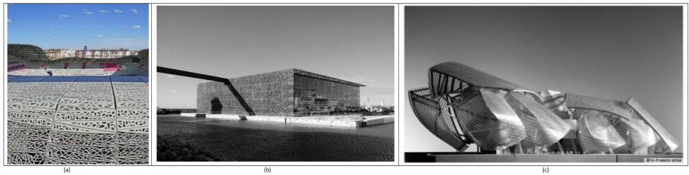
Figure 2.6 Architectural application of UHPC: (a) Jean Bouin stadium, France [62], (b) MUCEM, France [56], (c) Foundation Louis Vuitton, France [56].
