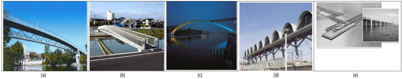
Figure 2.5 Structural application of UHPC: (a) Sherbrooke Footbridge, Canada [20], (b) Sakata- Mirai bridge, Japan [20], (c) Footbridge of peace, South Korea [20], (d) Roof structure of light rail station, Canada [61], (e) Haneda airport slab, Japan [56].
