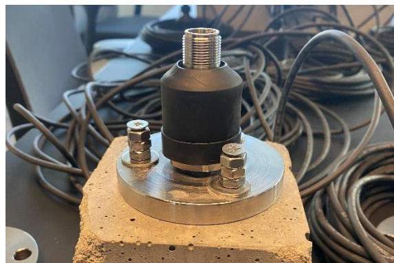
FIGURE 4: INSTALLED PLATE WITH ATTACHED SENSOR ON A TRIAL CONCRETE CUBE IN PREPARATION FOR THE REAL-LIFE INSTALLATION
