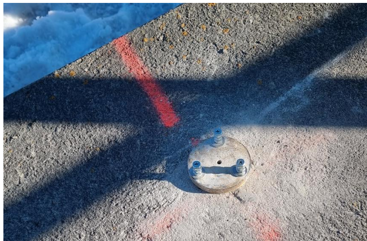
FIGURE 11: FULLY INSTALLED STEEL DISC ON THE WESTERN BRIDGE
