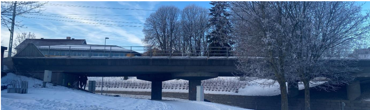
FIGURE 1: PICTURE OF THE EAST SIDE OF THE STANGE OVERPASS
