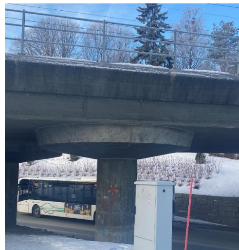
FIGURE 38: SOUTH COLUMN OF BRIDGE TWO OF THE STANGE OVERPASS
