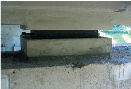
(a) Physical Example of an Elastomeric Bearing [29].
