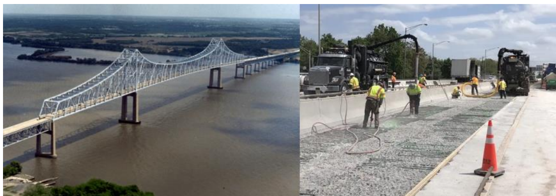
Figure 17 - L: Commodore Barry Bridge in Philadelphia [48] R: Removal of the old bridge deck [49]
