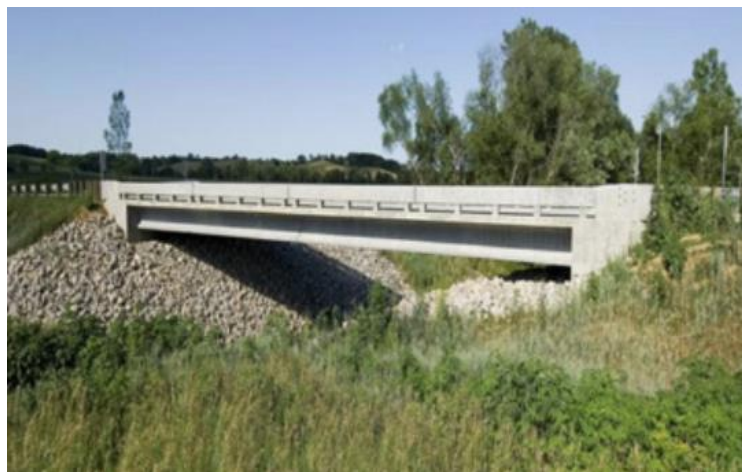
Figure 11 - The American Mars Hill Bridge [18]
