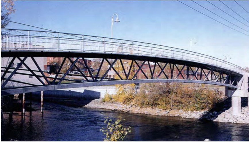
Figure 10 - Canada Sherbrooke Overpass [34]
