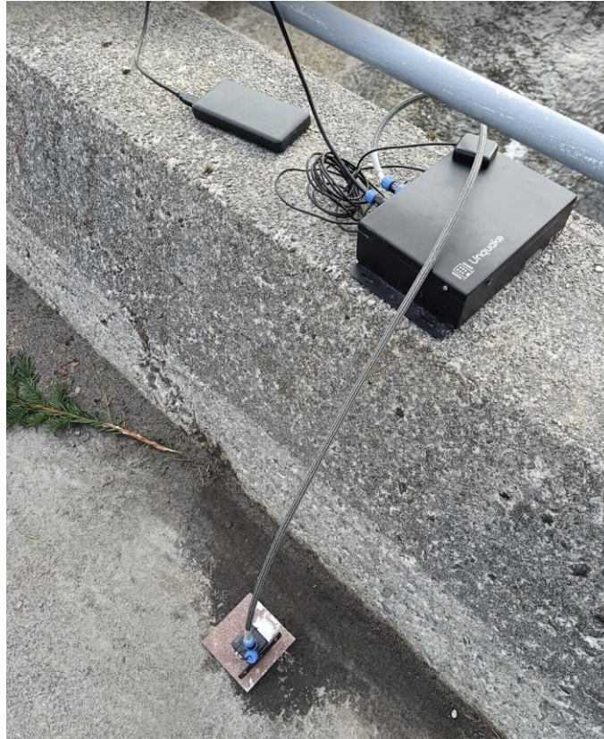
Figure 42 - Unquake OMAway sensor mounted on the Vattedal bridge
