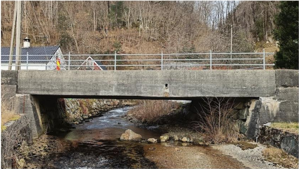
Figure 1 - The Vattedal bridge in Vestland County Municipality
