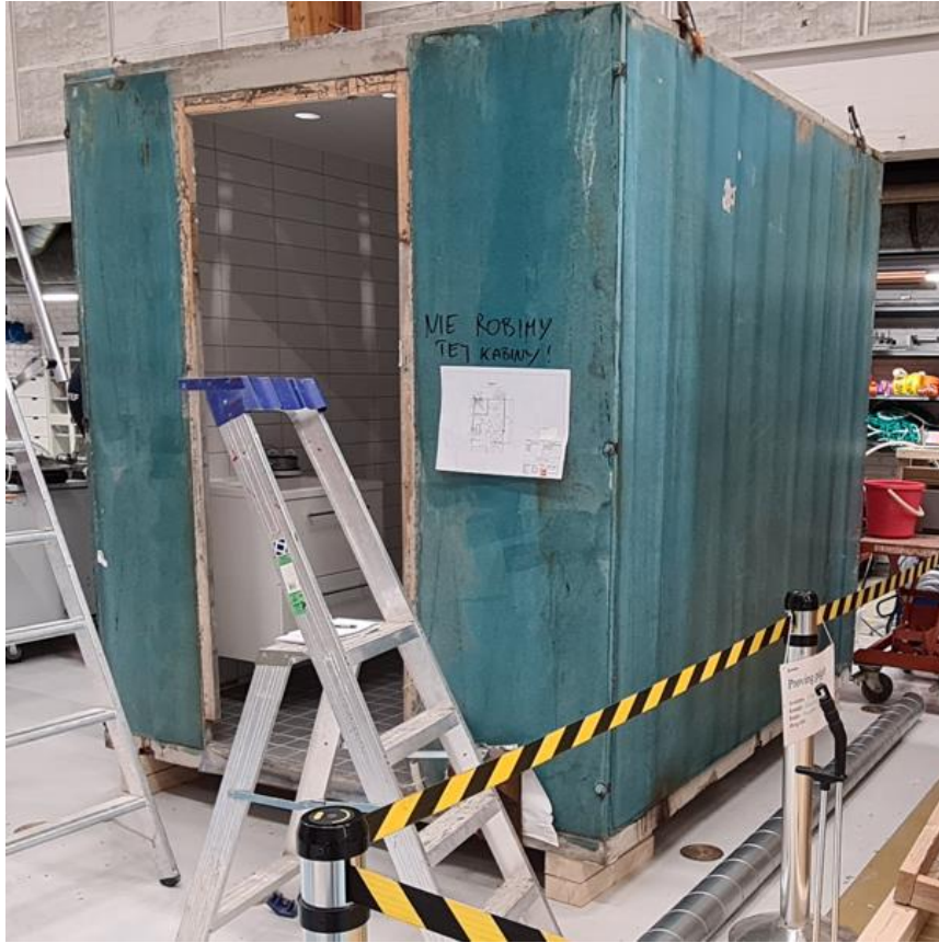
Figure 5: Outside view of the bathroom module before any work was done on it
