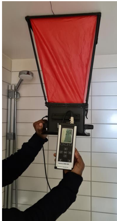
Figure 16: Swema air 300 measuring the ventilation over the shower space
