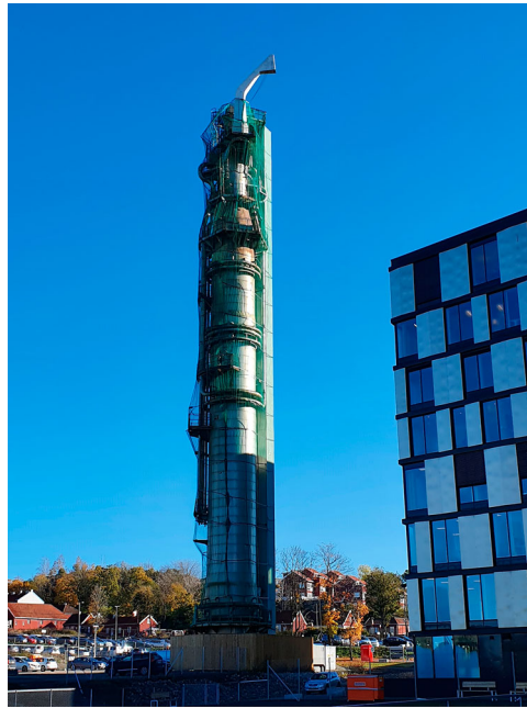
Figure 1. The digester. © Joar Skrede.
